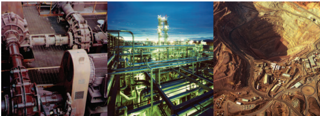
Maric valves control gland-water flow rate to three stage slurry pumping facility at Roxby Downs uranium mine South Australia"
